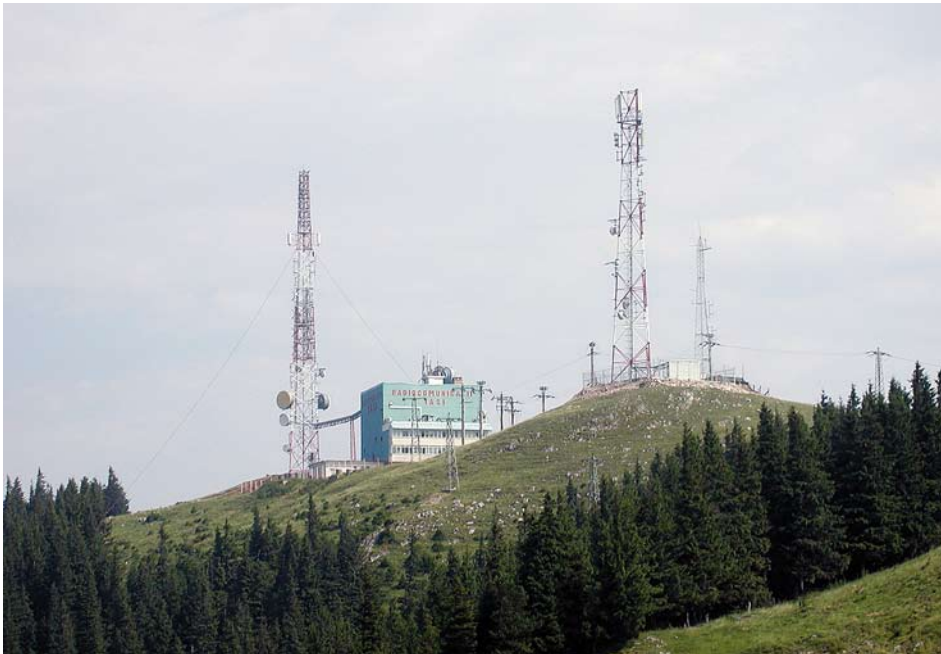
FIG 2 Antenna system at the Iași site in northeast Romania.
